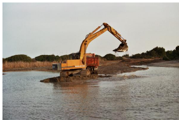
Works to restore one of the coastal lagoons (Author: Devesa-Albufera Service)
