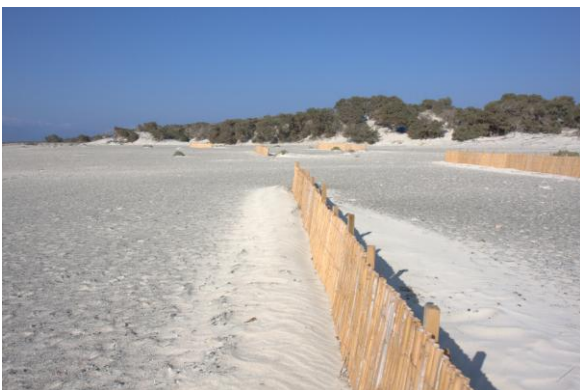
Sand trapping fences for the creation of embryonic dunes in Chrysi (Author: MAICh©)
