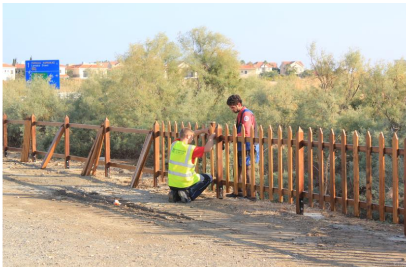
Fencing works (Author: M. Apostolidou©)
