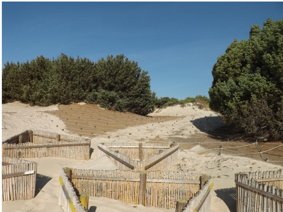
Environmental conservation at work: sand containment structures and coir mesh (Author: Martino Orrù)
