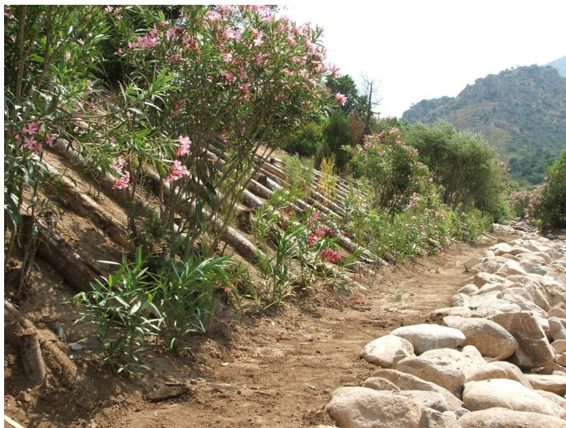
Site A: state of the art in September 2005 (Author: Enas)
