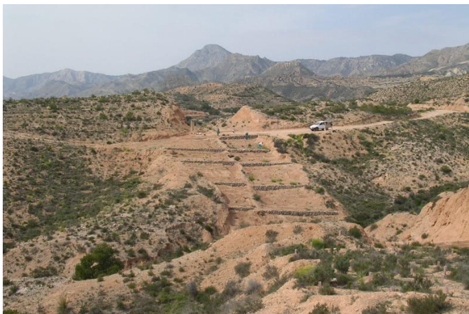
First steps in the restoration of the area affected by the pipe: adjusted slopes with little stone walls (Author: Alberto Vilagrosa)
