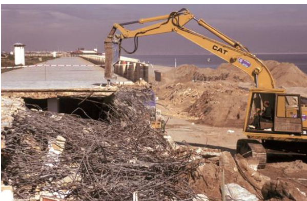
Demolition of past infrastructures (Author: Devesa-Albufera Service)
